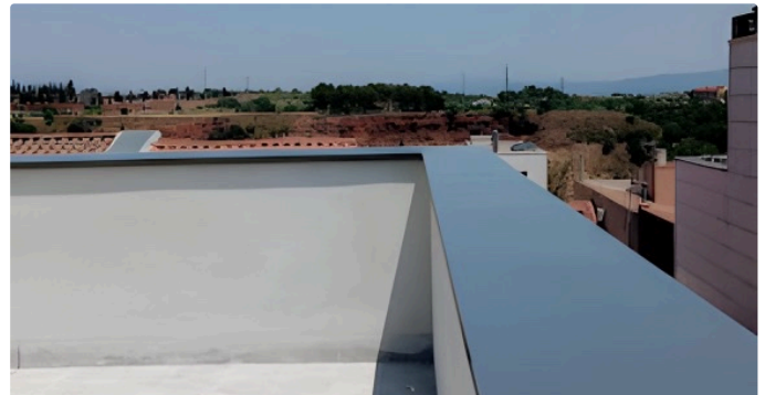
03 Continuous profile with no visible joints, RAL 7022
