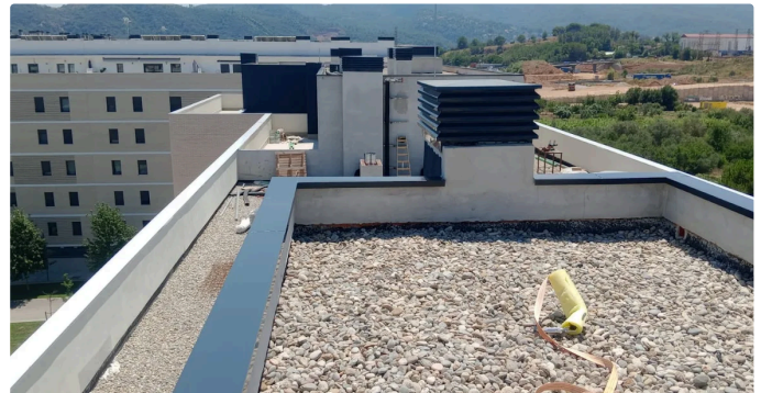
05 Residential building — ALU-CLICK® wall coping and VENTUM® chimney caps
